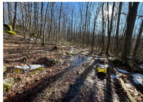
Ponding water indicates poor drainage
