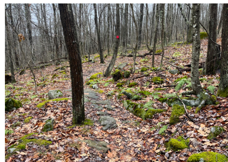
Rock armoring stabilizes tread to provide protection from erosion
