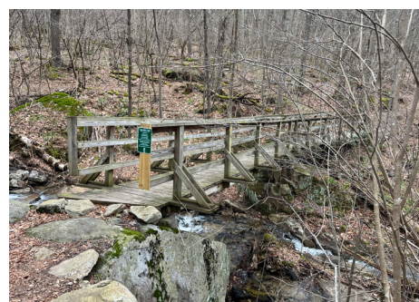
The bridge over Fork Run
