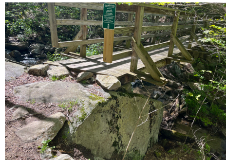
The bridge over Fork Run
