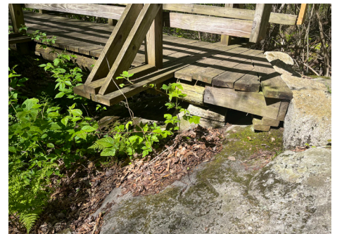
Abutments of the existing bridge crossing over Fork Run
