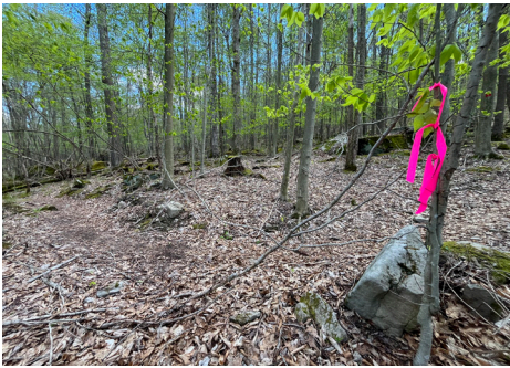
Examples of flagging at Fork Run. Triple flags indicate the beginning or end of a flagged segment, single flags represent corridor centerline, and double flags represent turns.
