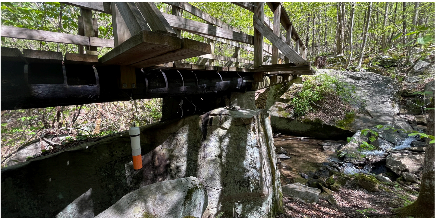
The existing bridge over Fork Run
